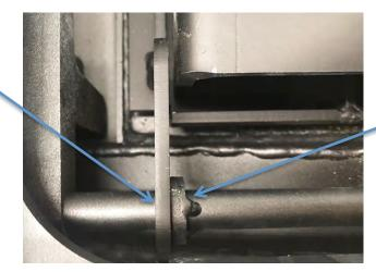
Welded bypass rod washer
