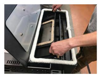
7. Leave the top lid open and lift the bypass handle up to the open position. Standing in front of the stove, the set screw that attaches the exterior bypass handle to the interior bypass rod will be found at the front right corner, inside the stove, under the top lid.
